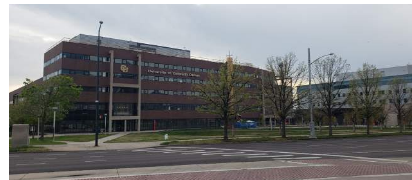
Site from Speer Boulevard and Lawrence Street
