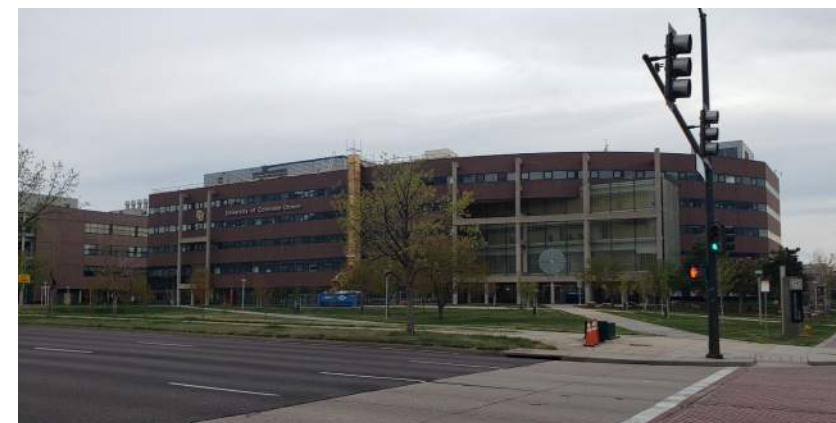
Site from Speer Boulevard and Larimer Street
