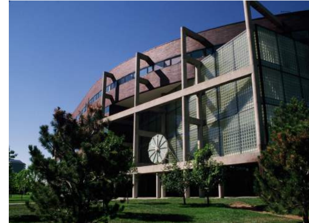
North Classroom Building
