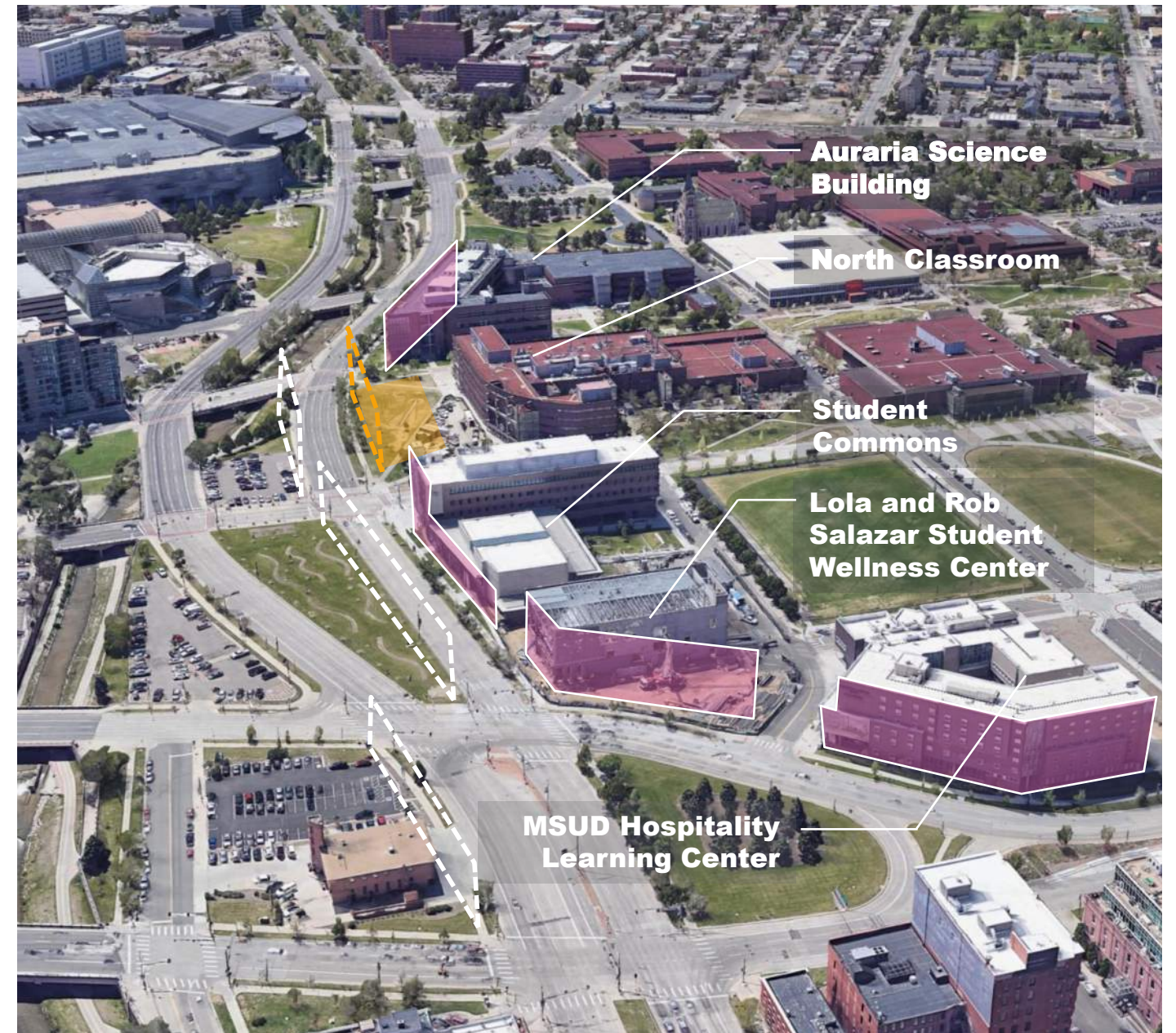
Aerial Image - Speer Boulevard Facades
