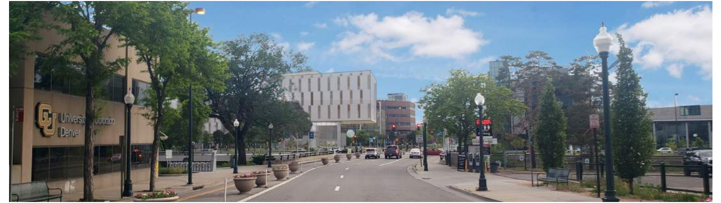
View from Larimer Square to new CEDC Building, new plaza, and North Classroom clock beyond
