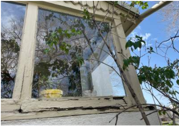
North facing wood windows at rear addition. Severe deterioration at the window sill and lower portion of the frame.
