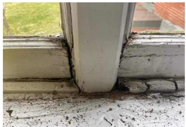
Water damage at the window mullion.
