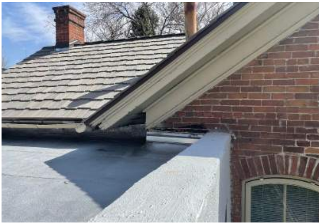
Parapet and flat roof at rear addition, synthetic shingle roofing.
