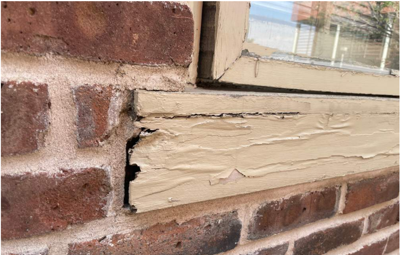
Wood sill deterioration and paint delamination from water infiltration.
