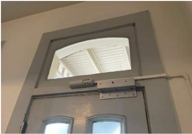
Transom and request to exit door hardware at the main entry door.
