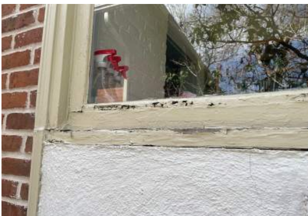
Deterioration of the wood window and sill at the north elevation of the rear addition.
