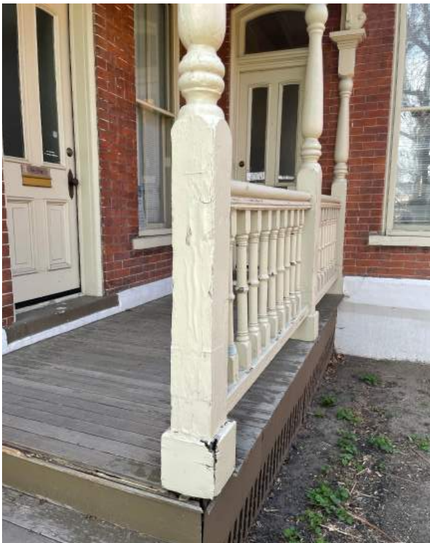
Water damage resulting in deterioration of the paint at turned porch columns and wood at the column base.
