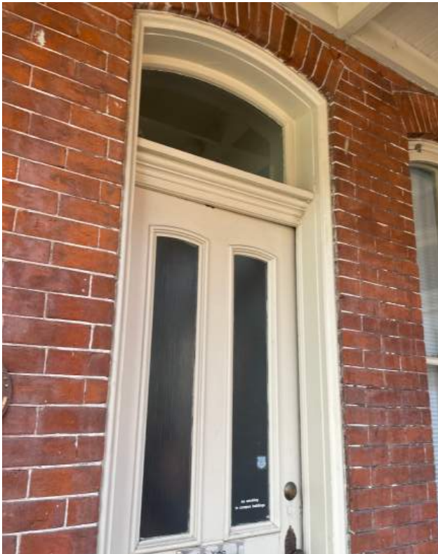
Secondary paneled wood entry door and transom window.
