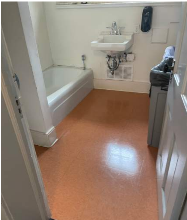
VCT flooring in the existing Bathroom.
