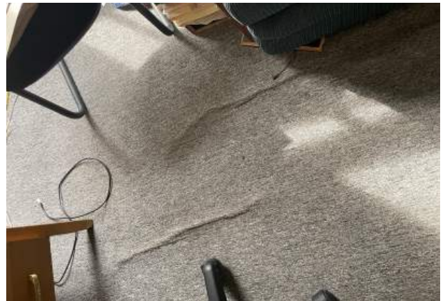
Carpet in existing Office 2 is stretched and wrinkling.
