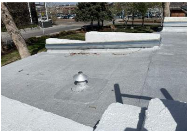
Plumbing vent over the bathroom.
