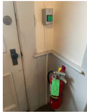
Push to exit door hardware at main entry door.
