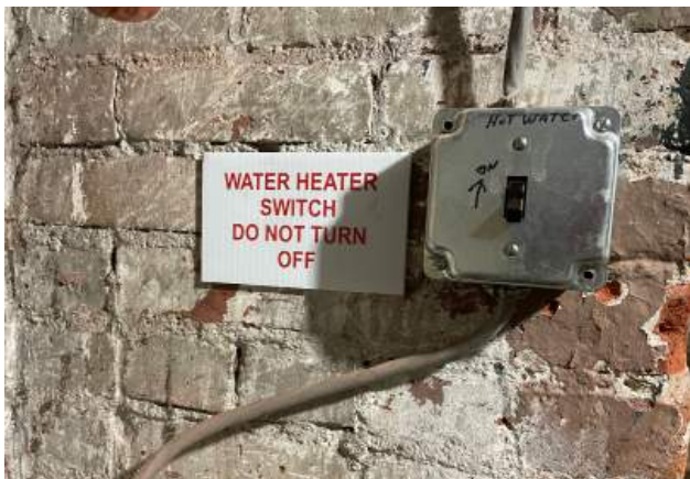
Water heater switch.
