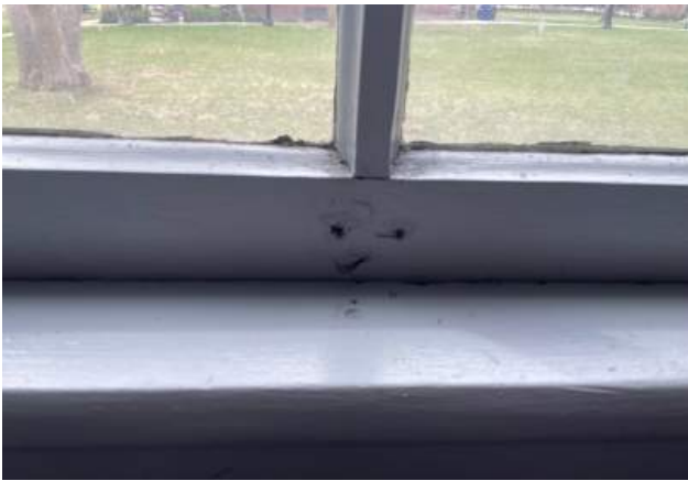
Missing hardware at bottom sash of existing window.
