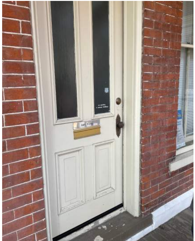
Secondary paneled wood entry door and transom window.
