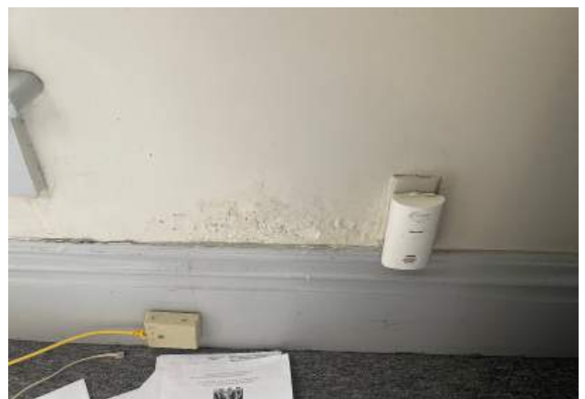
Plaster damage at south wall of existing Office 2.
