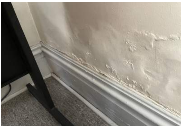
Plaster and paint damage at base of south wall.
