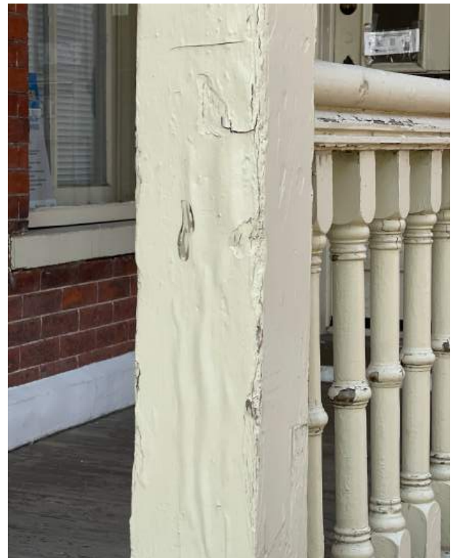
Paint bubbling at porch column.
