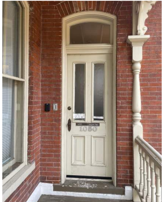
Paneled wood entry door and transom window.
