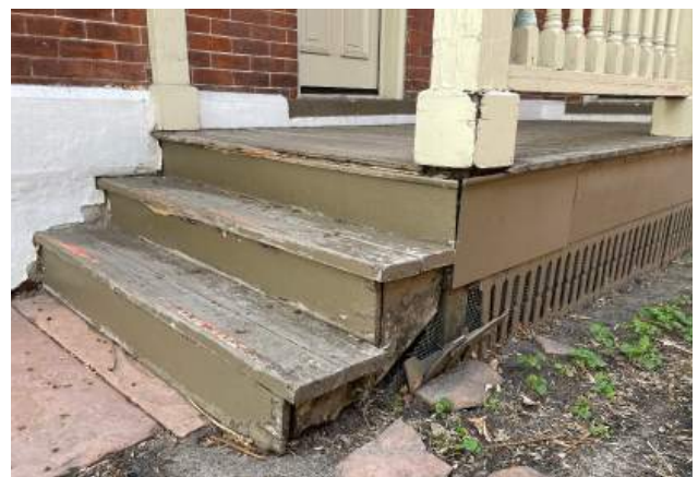
Wood stringer, floor structure, and screening material.
