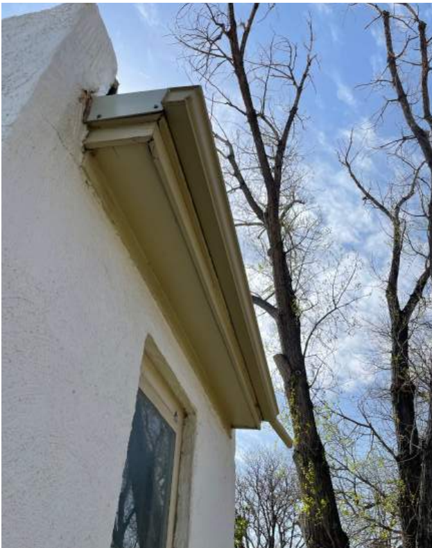
Gutter and downspout at west elevation of rear addition.
