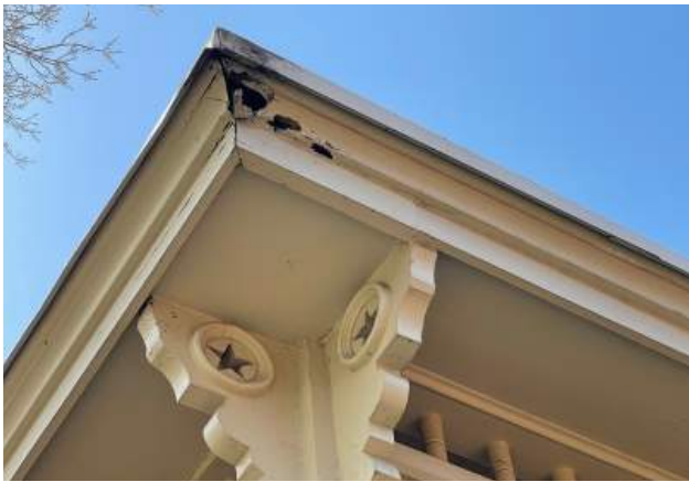
Fascia damage at porch roof corner.
