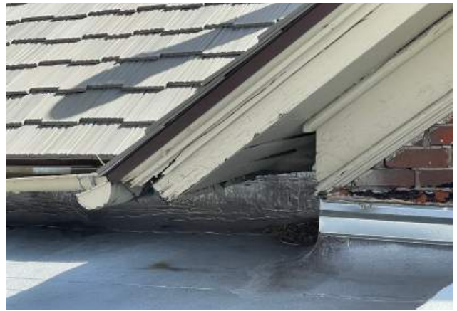
Deterioration at the wood fascia and eaves overlapping the flat roof.
