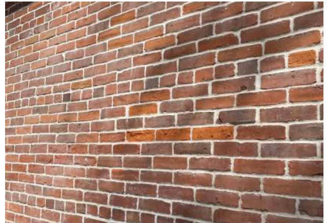
Condition of red brick at the south elevation. Common bond pattern.
