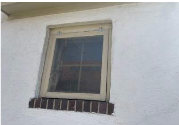
Wood window with storm and a brick sill at the west elevation.
