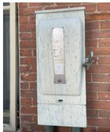
3 Phase, 240 volt, 200 amp electrical panel.
