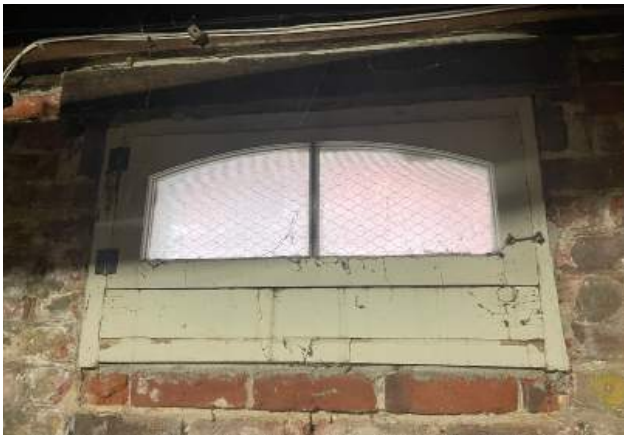
Original wood window with wire glass.
