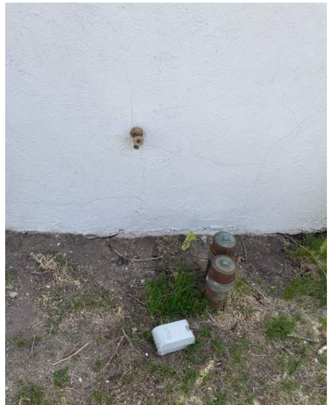
Hose bib and access to waste line?
