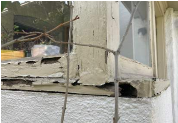
Severe deterioration at the corner of the wood window/sill.
