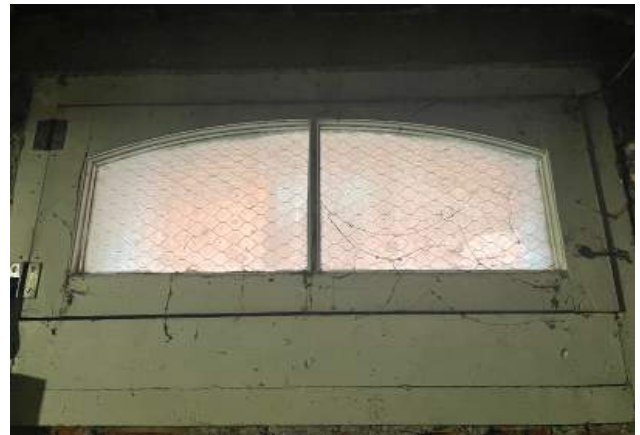
Original wood window with wire glass.
