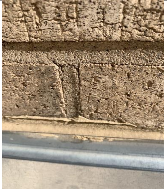
Description: Yellow Parapet Wall Flashing Caulk (CK1)
