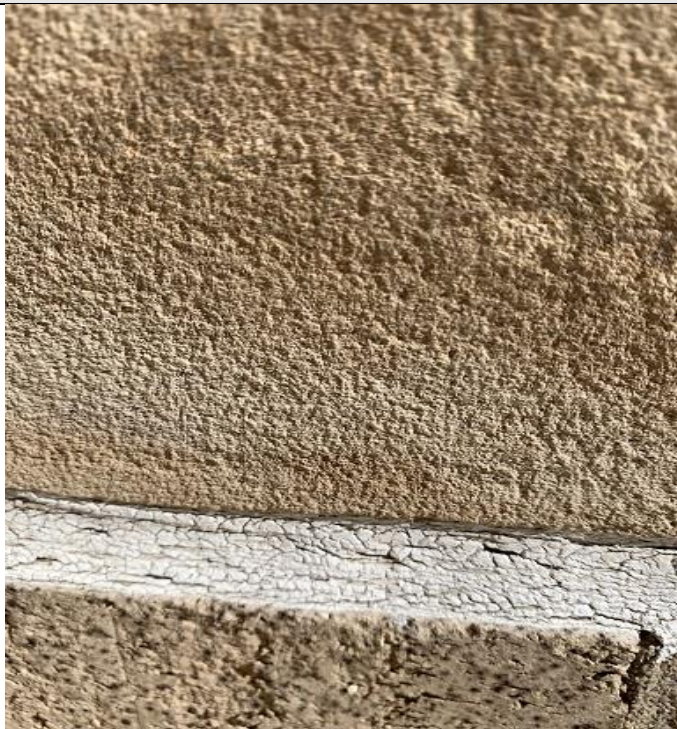
Description: White/Grey Parapet Wall Caulking (CK2)
